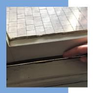
Both types come in different widths and styles - you may have to experiment with these to find the right size for your door or window. You can buy a few different sizes to see which works best. You'll know it's right when the stripping creates a tight seal, leaves no gaps and compresses very slightly between the door and the door frame. For large gaps, you might need to stick additional layers of tape over the first layer.
