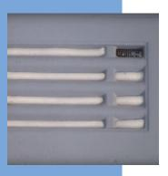
**TIPS:** This technique can be used for all different kinds of wall vents - just cut the gap filler rod to match the shape of the vent (see 4th image for an example). Gap filler rod can be removed in summer to allow for better ventilation.
