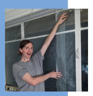
**TIPS:** If the bubble wrap isn't sticking in certain places, just respray the window with water. If the sheet falls down, try cleaning the window thoroughly and repeating the process. You can also secure the bubble wrap with some sticky tape at the edges of the window.
