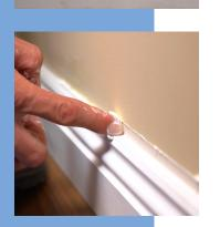
**TIPS:** If the gaps are large, you can fill them with gap filler rod (Moroday, \$5-10, available in different diameters at Bunnings) before caulking simply push appropriately sized rods into the gaps to achieve a tight fit and cut to length. Top these with sealant.
